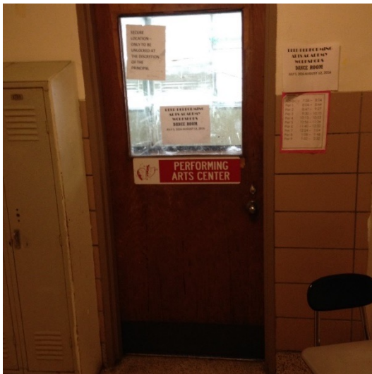
Existing Classroom Doors
