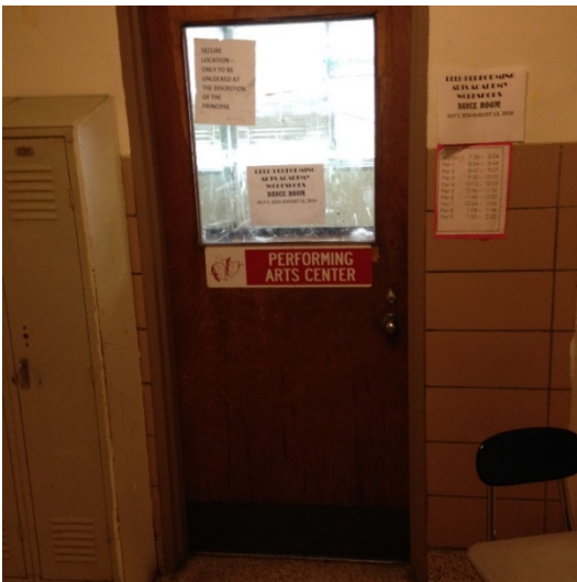
Existing Classroom Doors
