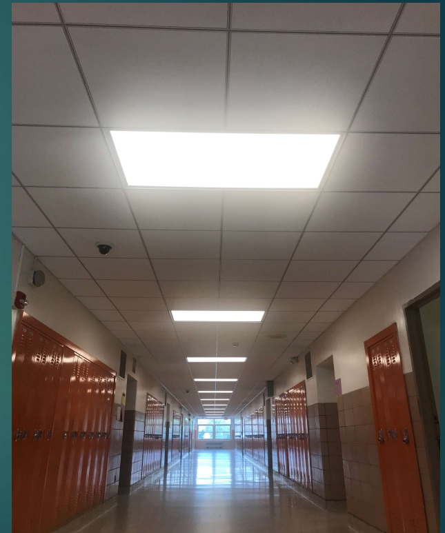
New Drop Ceilings with Lay-In LED Lights
