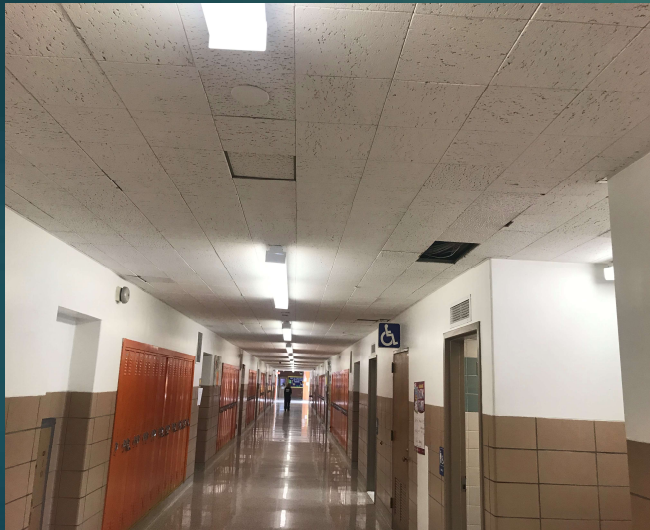
Old Spline Ceilings with Surface Mounted Lights
